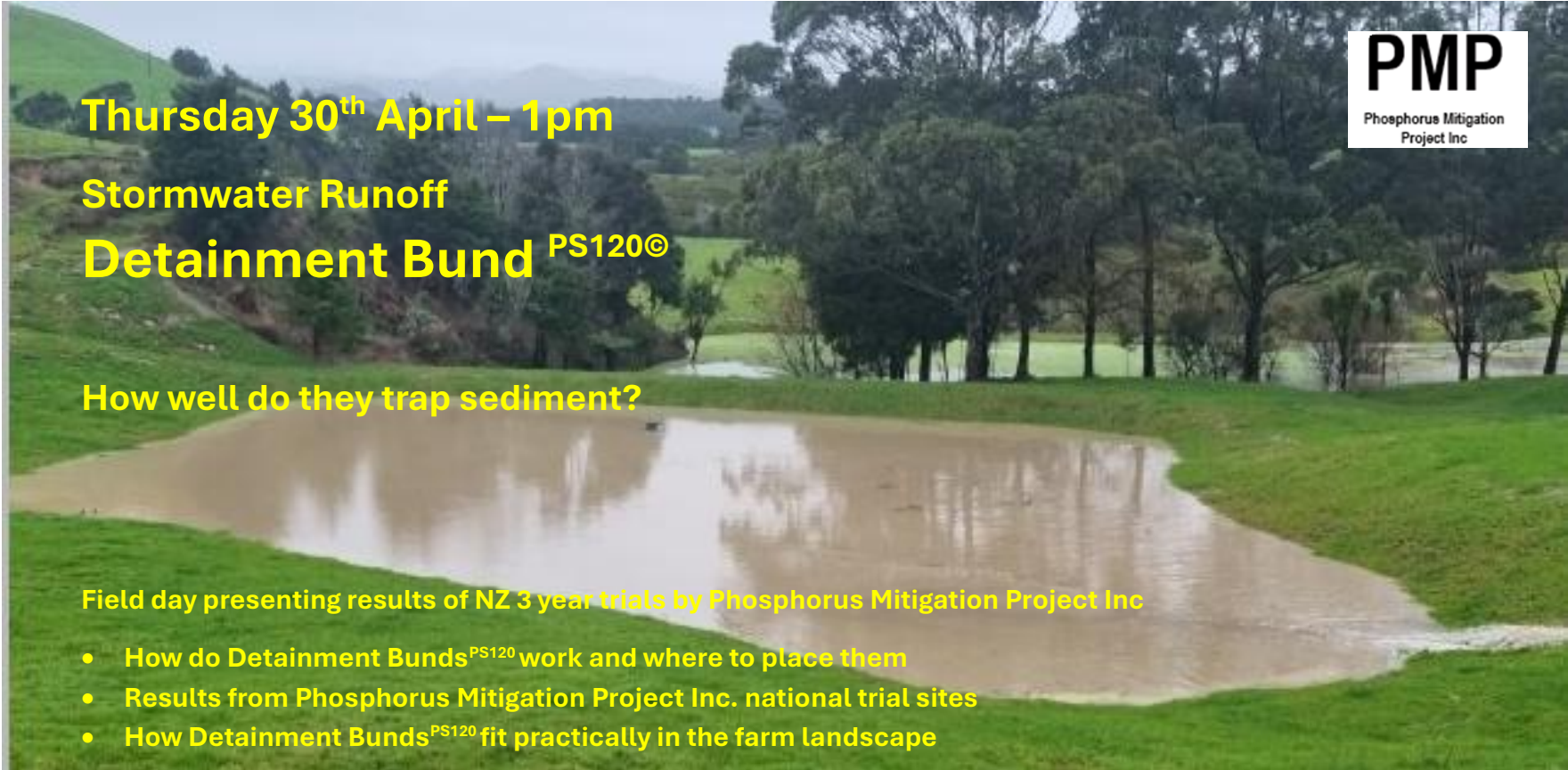
A full and functioning Detainment Bund PS120 during run-off event July 2022, Kuwara Trust Farm.
